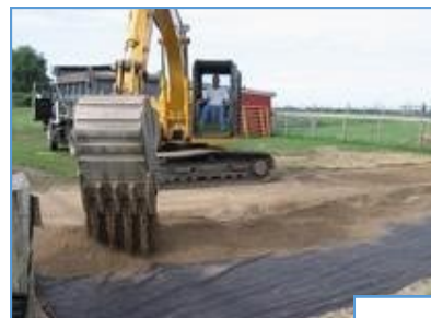
Left: Geo-textile fabric separating natural soil and 6-8 inches of process sand and gravel (top footing).
