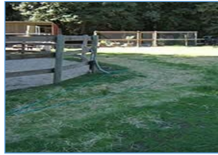
Grass swale intercepts runoff from surrounding land and diverts around the livestock yard. Photo courtesy of the Livestock and Land Program, CA.
