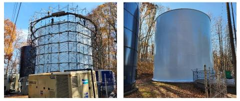
wall hatch, overflow pipe, ladders and a roof safety climb system; replacement of platform gratings; modifications to the roof vent; and coating the concrete foundation for a cost of \$716,249.78. The work performed will extend the life expectancy of the tank for 25 years.
