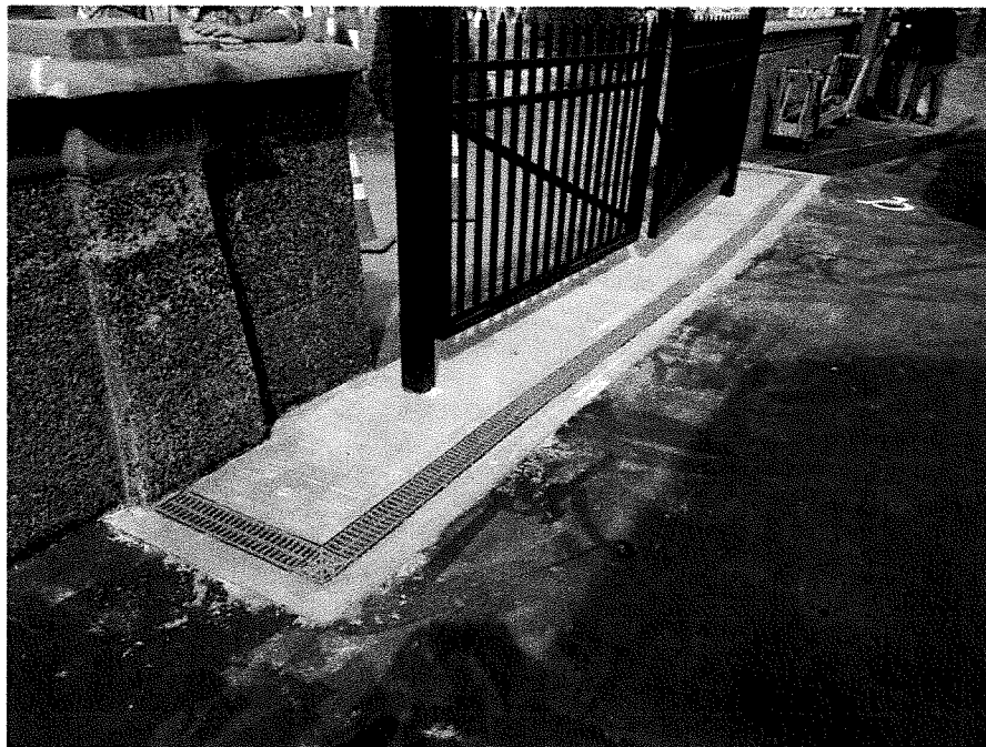
Photo 1 – Trench Drain at Connecting Driveway
