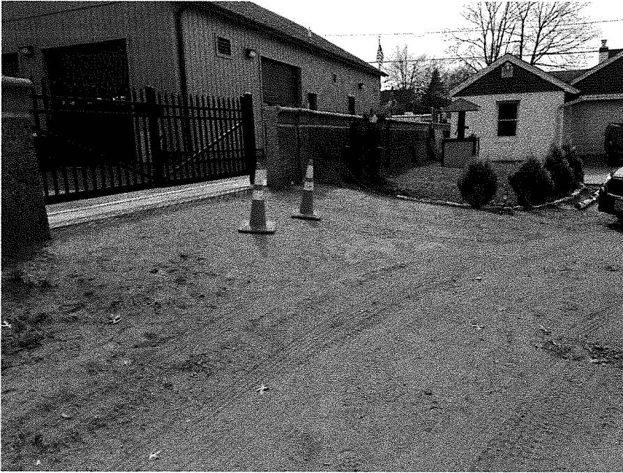
Photo 2 – Re-Graded Connecting Driveway
