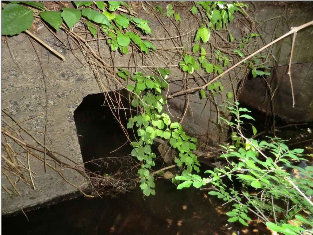
Photo 1: Culvert Inlet
