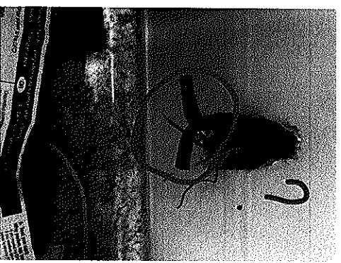
Old bad wiring found when changing out outlet, no ground, No junction box in attic, just electrical Taped.
